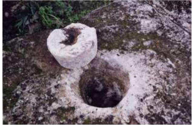
Vertical holes in pipes only had to be tightly sealed where inside pressure head was higher than atmospheric pressure. Small pressures were also at the beginning and sometimes at the end of a discharge pipe. There, the cover could be leaking. Holes in water pipes may also have had other functions. Not every hole can be regarded as air chamber to avoid water hammer damage.
