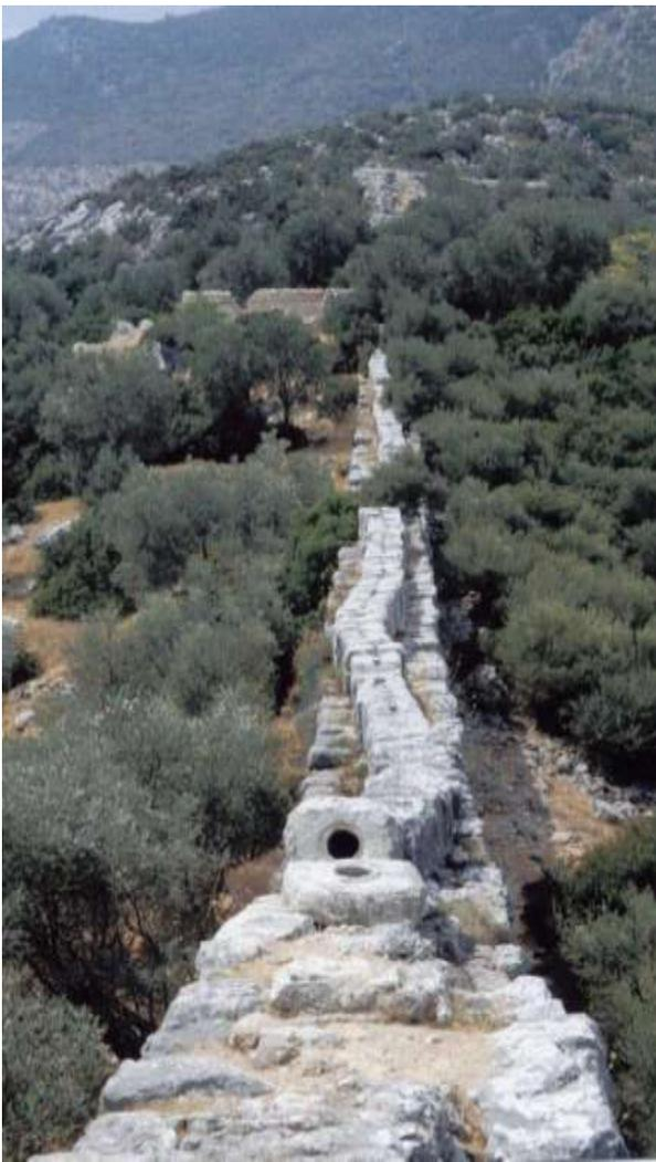
In operation, the holes were closed by branching tubes, by covers or by bungs.
